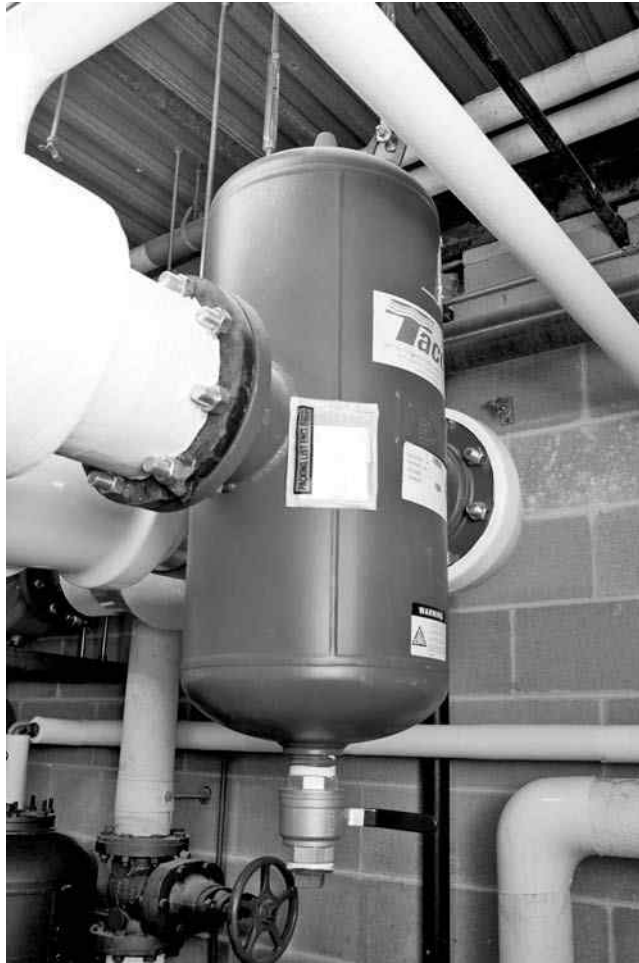
FIGURE 10-20 Taco 4900 microbubble air separator.
