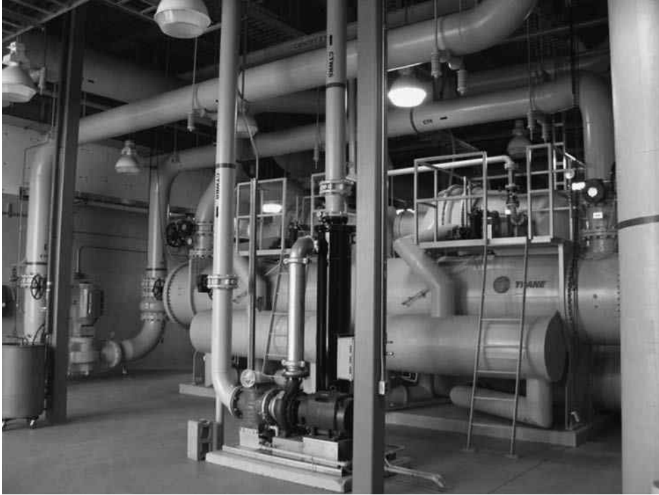
FIGURE 4-16 Chillers can be designed to be reverse cycle, just as a heat pump has a reverse cycle. In this case, the chiller can provide heated water, similar to a boiler, at a coefficient of performance (COP) approaching 5.0. ( Trane. )
