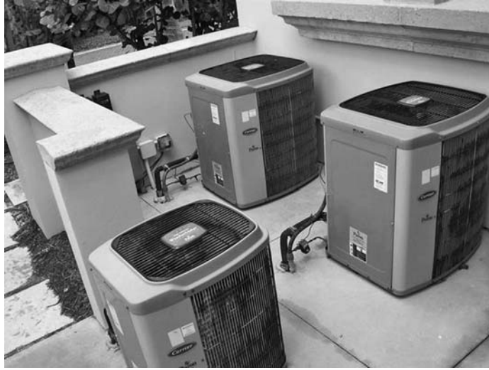
FIGURE 1-4 These air-cooled condensers are significantly weathered after only 4 years of exposure to the elements. This type of weathering is all but eliminated when the equipment is brought indoors, as in geothermal applications. ( EggGeothermal. )
