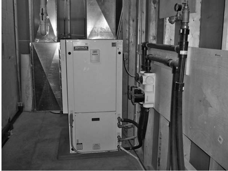
FIGURE 3-19 A two-speed high-efficiency geothermal system with electronically controlled motor two-speed compressor. Today's geothermal heat-pump equipment needs smart controllers. With the introduction of direct-current (dc) inverter-driven variable-speed equipment, this is more important now than ever. ( Geofinity. )
