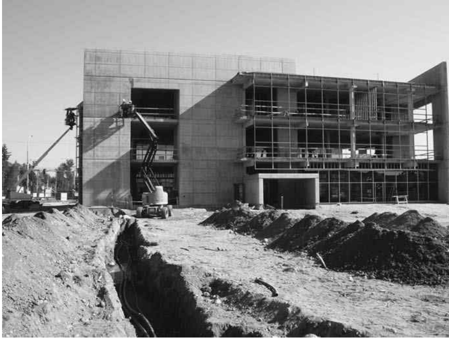
FIGURE 4-9 Placing a geothermal closed-loop exchanger under a parking lot works especially well with the lithology is mostly rock. ( David Hoffman. )
