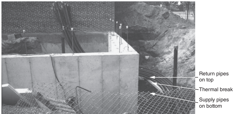
FIGURE 7-17 Use of HDPE or underground connections provides for worry-free installation, provided that accepted industry practices are followed. Note that the HDPE also exhibits a greater tolerance to wide variations in temperature. ( Water Energy Distributors. )
