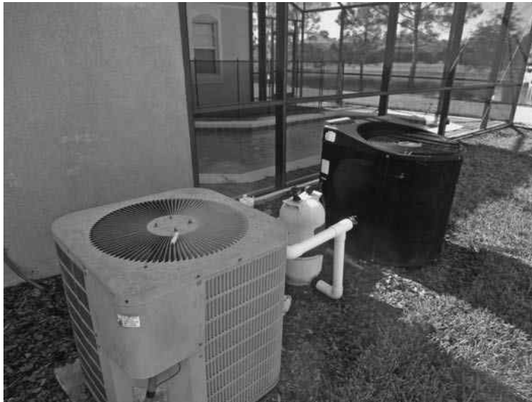
FIGURE 13-6 These two heat pumps doing their job side by side for the same dwelling could be likened to the old adage, “One person’s trash is another person’s treasure.” Much energy is expended in an effort to remove heat (for the building), while much energy is also expended in an effort to bring in the heat to the pool. ( EggGeothermal. )
