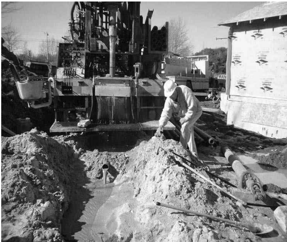
FIGURE 7-8 The well driller will sample rock cuttings during the process of drilling. (Water Energy Distributors.)
