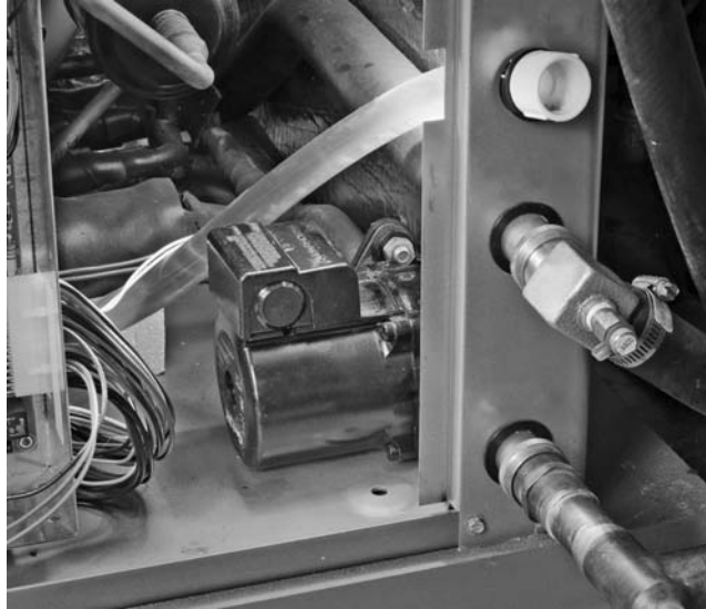
FIGURE 2-2 Anytime you can integrate factory-installed options into the packaged equipment, you will reduce field mistakes. Additionally, factory-installed pumps, valves, and controls have been proven to reduce energy consumption over field-installed hydronic specialties. (WaterFurnace.)
