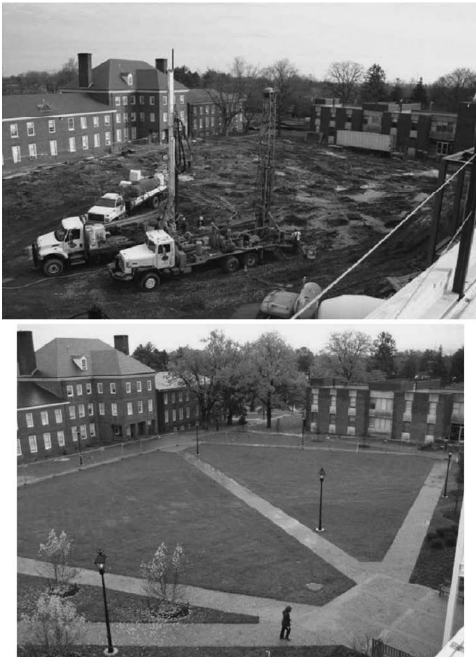
FIGURE 4-8 It is evident in these before and after photos of the geothermal loop field placed in the courtyard of Washington College that there will be little chance for damage of the loops by future activity. ( David Hoffman. )
