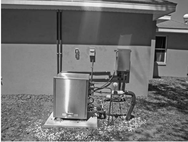
FIGURE 2-9 This direct-exchange GHP system, installed in Kissimmee, Florida, uses a copper exchanger and contains refrigerant that provides the heat exchange necessary for the cooling and heating of the residences in the development. Although the condenser is placed outside, it also could be placed inside the structure because it requires no condenser fan ventilation. (EggGeothermal.)
