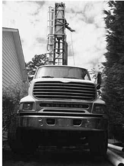
FIGURE 4-10 As seen here, drilling can be rather invasive. Logistically, it is important to make sure that the equipment needed to perform the job can gain access. Once the driller is done, the landscaping is replaced, and everything is back to normal. ( EggGeothermal. )
