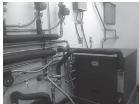
Water to Water (Spectrum Equip)
