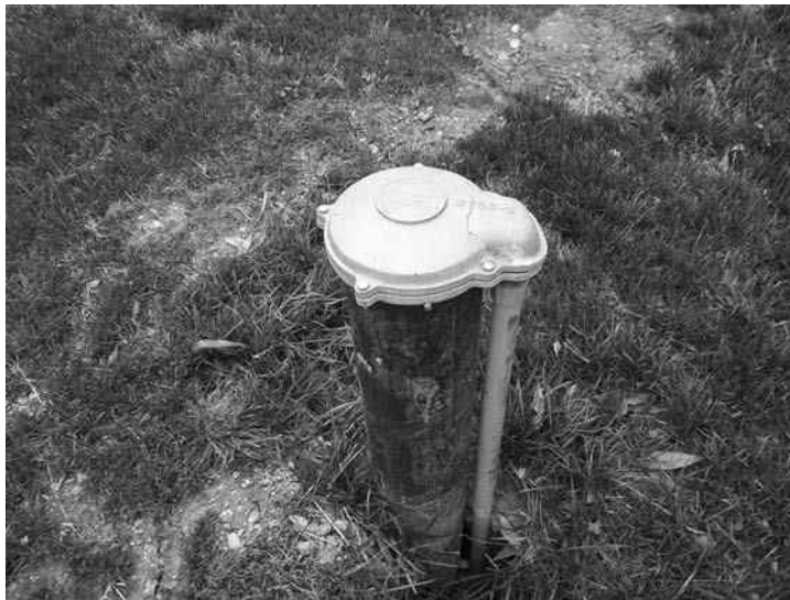
FIGURE 3-31 This is the actual 1500-ft-deep standing-column well installed at the Riversdale Museum in Delaware, along with some of the equipment and piping installed in the service the structure. If this were a closed-loop well, it would provide about 6 tons of heating and cooling capacity. Instead, the capacity is about five times that. ( EggGeothermal. )
