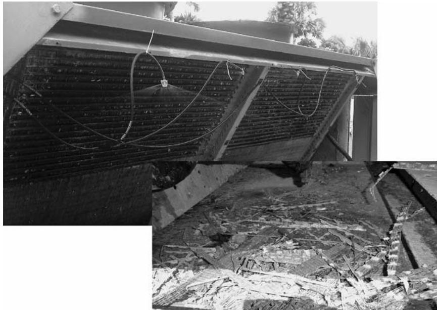
FIGURE 1-5 The aluminum fins that were formerly attached to this condenser's copper piping have separated and fallen to the ground. Long before condenser fins actually fall off the refrigerant piping, the capillary bond between the aluminum and the copper oxidizes and creates a type of insulation, significantly reducing efficiency. ( EggGeothermal. )
