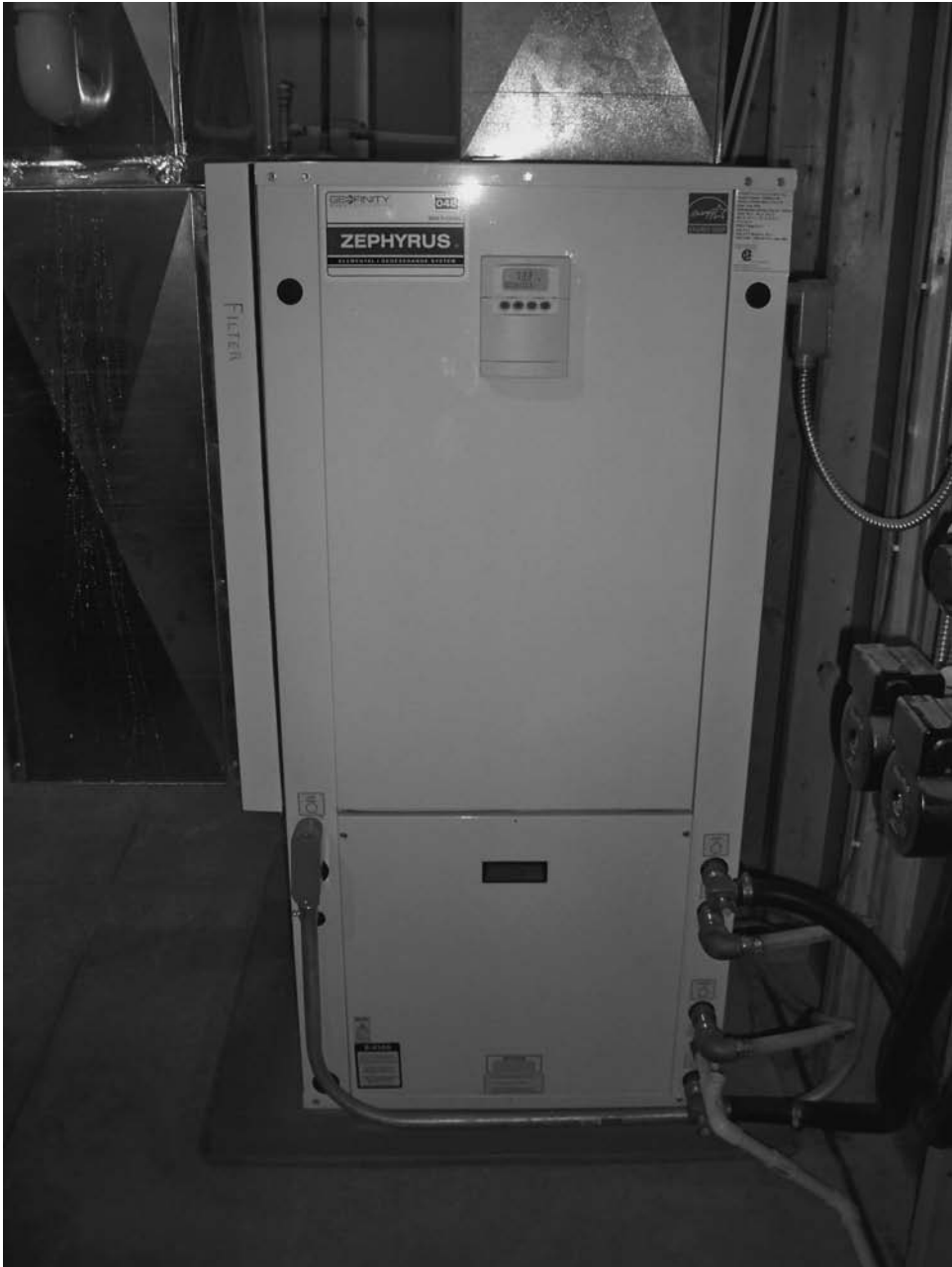
FIGURE 4-19 Elegant and simple. A unitary geothermal heat pump contains all the necessary components to provide domestic hot-water heating and air-conditioning, as well as in some cases pool or spa heating. This is the essence of simplicity—load-sharing, load-shedding sustainable and effective design. ( Jacobs Heating. )
