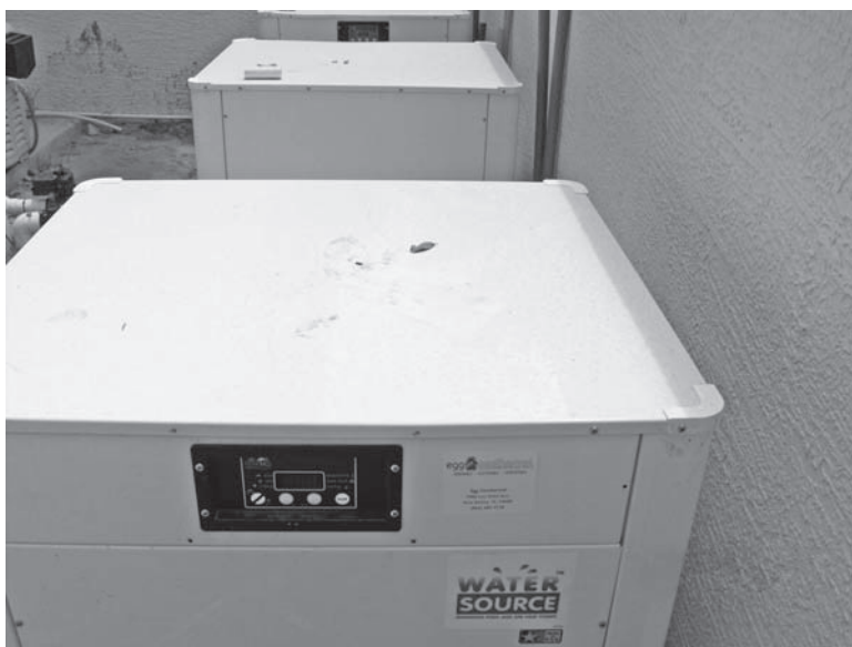
FIGURE 1-3 Geothermal heat pumps provide a fundamentally limitless source of heat for the purpose of pool heating at efficiencies that are not attainable by any other regularly used technology. (a) A geothermal heated pool. (b) The pool heat pump. (EggGeothermal.)
