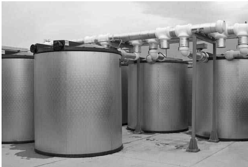
FIGURE 9-10 An ice-bank thermal storage tank.
