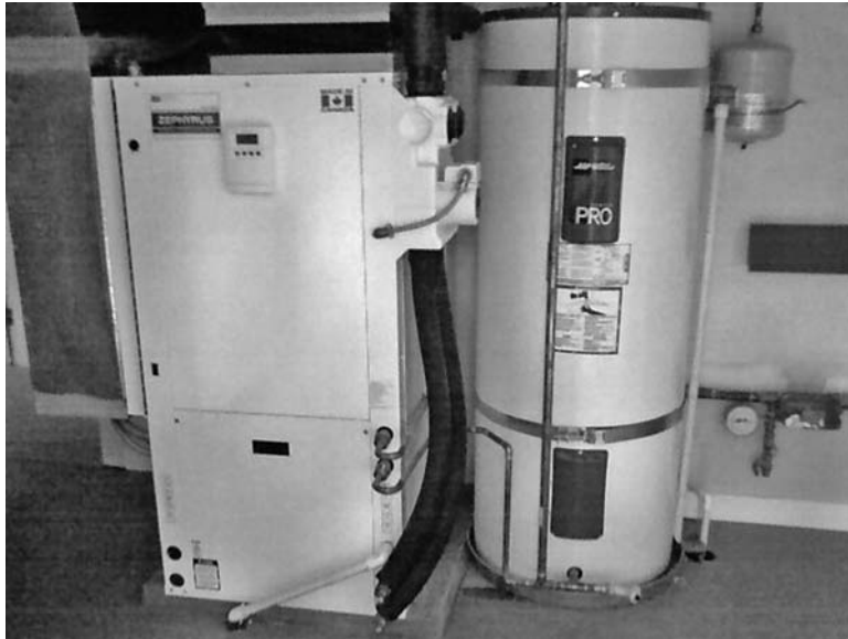
FIGURE 1-7 High-quality products such as this Geofinity GHP are available with options such as on-demand domestic hot-water generation and are highly desired by customers. As with any industry, engineered failure may begin to creep in, and designers must be vigilant to keep the best interests of their customers at heart. Be careful in your equipment selection and choice. (Geofinity.)
