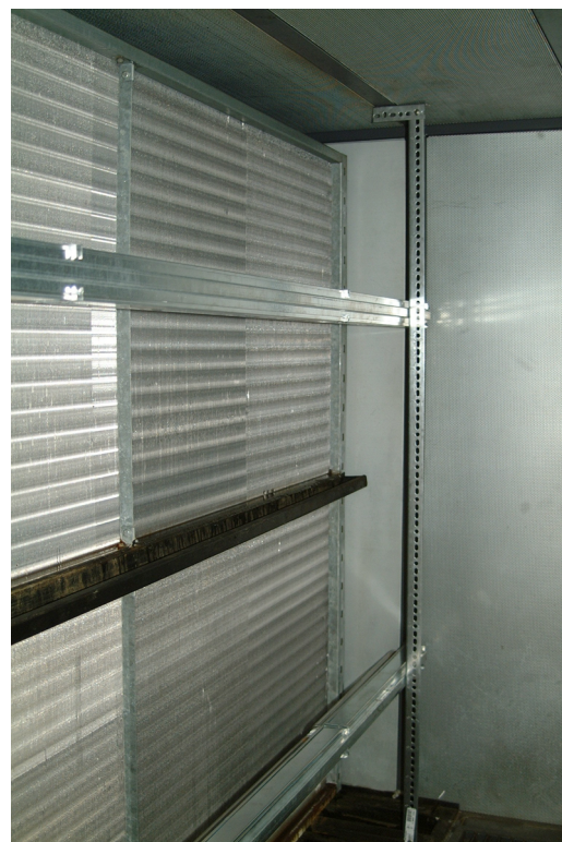
Fig. 8 Horizontal Lamp Placement for Coil Surface Disinfection
