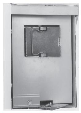
Figure 6-7 Disconnect switch used for air conditioning equipment. (Source: Delmar/Cengage Learning)
