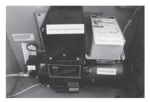
Figure 39–8 Oil burner assembly with pump, burner motor, primary control, and ignition transformer. (Source: Delmar/ Cengage Learning)
