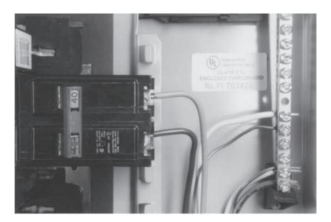
Figure 5–19 240-volt single-phase threewire connection. (Source: Delmar/ Cengage Learning)
