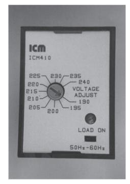
Figure 36-14B Voltage adjustment for the three-phase line monitor. (Source: Delmar/Cengage Learning)
