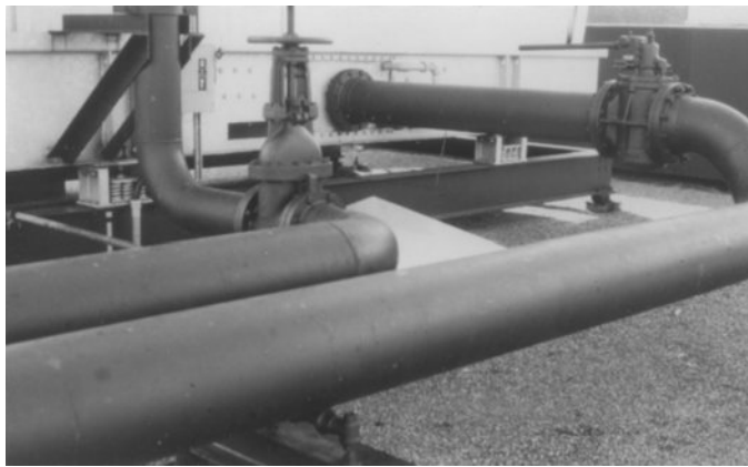
Figure 8-18 Incomplete vibration isolation at cooling tower. Even though the tower is isolated, the condenser water pipe supports are mounted rigidly to the roof. This allows some tower vibration to enter the roof structure.
