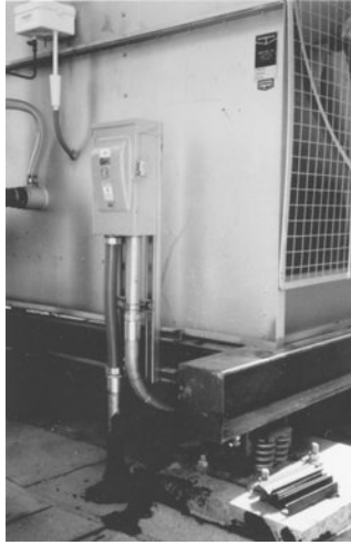
Figure 7-9 Taut outdoor “flexible” conduit forms a vibration “short-circuit” at cooling tower. The grillage under the cooling tower is resting on spring isolators, but the short conduit between the disconnect and the roof penetration transmits tower vibration into the roof.
