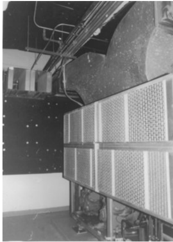
Figure 8-8 Proper installation of an indoor self-contained packaged HVAC unit. Note the dual radius supply duct split on top of the unit; the return air sound traps to the left of the supply duct, the black plenum liner on the mechanical room wall, and the spring isolator under the unit.
