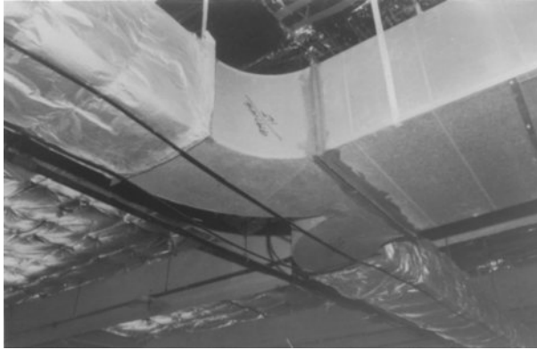
Figure 8-13 Duct split using radius elbows. This design is preferred because it produces less pressure drop and noise than a bullhead tee.
