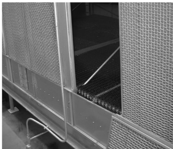
Figure 3-9 Honeycomb water basin silencers installed several centimeters above the water surface to reduce the velocity of the falling water before it hits the basin.
