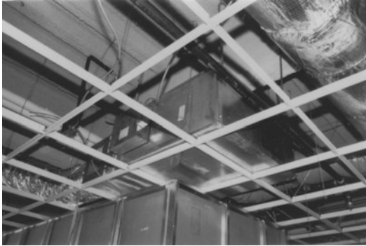
Figure 8-7 Improperly installed fan-powered variable-air-volume unit. The unit is resting on the ceiling grid. This allows unit vibration to transmit directly into the partition below. The partition then acts as a sounding board, radiating noise into the occupied space.
