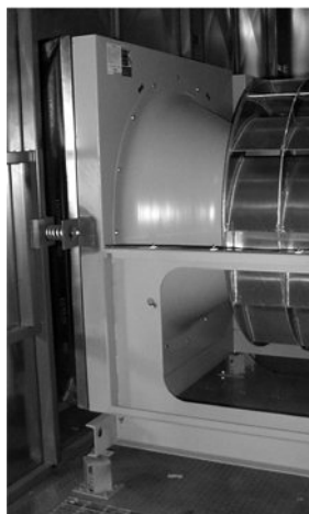
Figure 5-9 Thrust restraint at mid-height of fan inlet panel prevents contact between the panel and the equipment housing framework. An identical restraint is installed on the opposite side of the fan.
