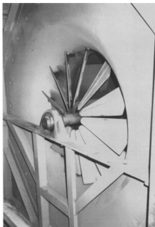
Figure 2-51 Nested inlet vanes obstruct airflow.
