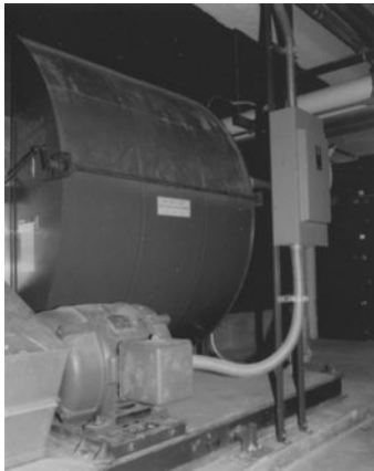
Figure 8-20 Correctly installed flexible conduit between electrical disconnect and motor. The flexible installation reduces fan and motor vibration in the floor slab.
