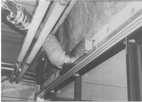
Figure 2-25 Poor inlet duct connection to a supply air ceiling diffuser. The winding flex duct path causes excessive air turbulence and noise at the diffuser's inlet collar. This diffuser could produce noise levels as much as 15 dB higher than the manufacturer's catalog data.
