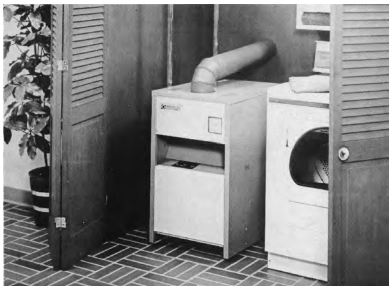
Figure 9-1 Electric-fired boiler. (Courtesy National Better Heating-Cooling Council)
